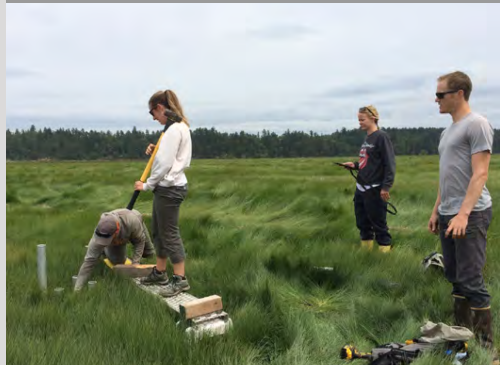
Installing Surface Elevation Table platform at Nanaimo River estuary
