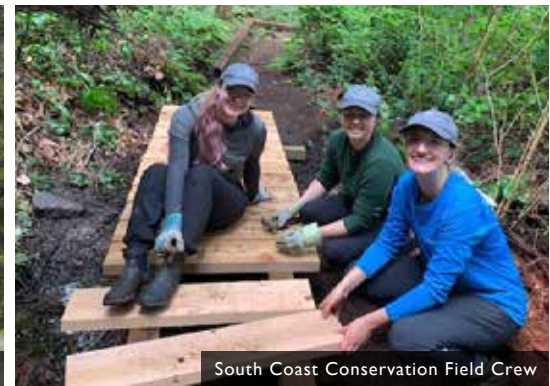
South Coast Conservation Field Crew
