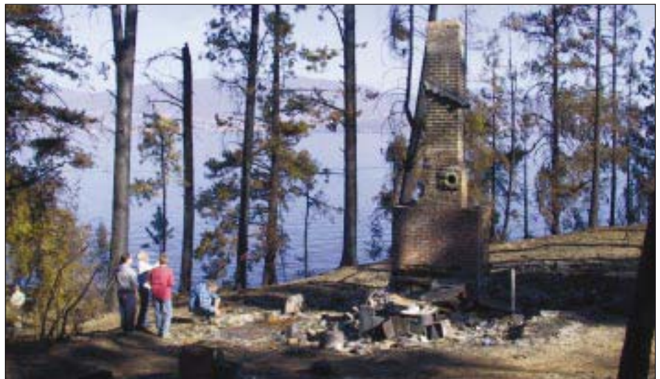
Assessing fire damage at Okanagan Mountain Park, Kelowna
